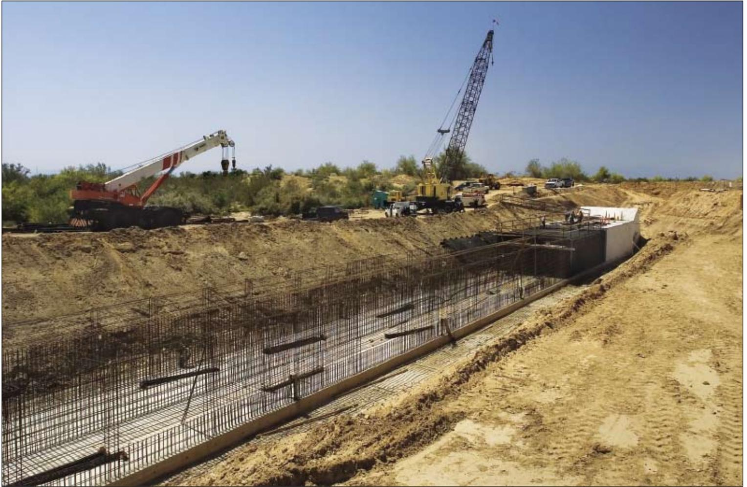
**The last portion of the Coachella Canal to remain earthen is being lined with concrete to reduce water lost due to seepage. This massive project is expected to cost \$83.6 million, including \$71 million for construction alone.**
