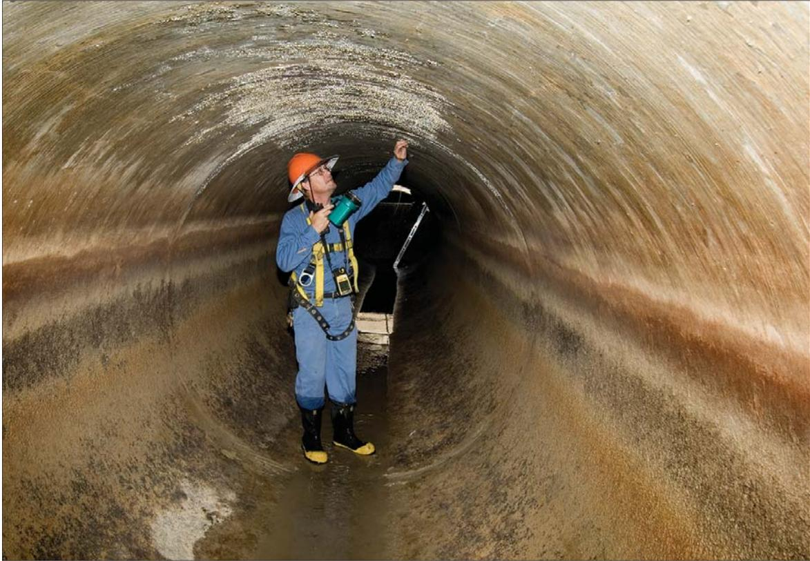
Crew Chief Rod Nason, a 21-year employee, conducts a routine inspection of a large lateral pipe used to deliver Colorado River water from the Coachella Canal to area farms. These inspections, which require temporarily shutting down the water supply to allow employees to safely enter, are the perfect time to check for the existence of quagga mussels. To date, none have been found in CVWD's system.
