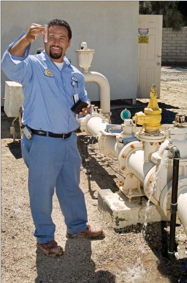
Paul Zepeda, a domestic water service worker, takes a water sample from a CVWD well to perform a routine on-site test of the water's chlorine level.
