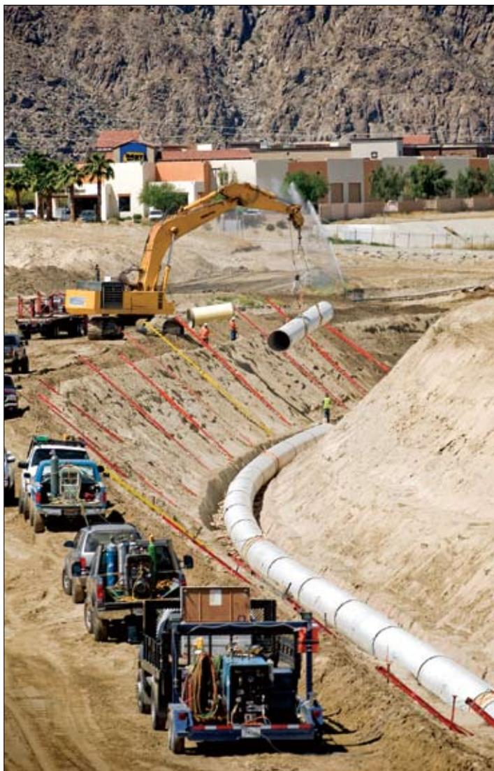
Left: While being constructed in the Whitewater and Coachella Valley Stormwater Channels, the 54-inch steel pipeline could be seen from roads and bridges crossing the channels.
